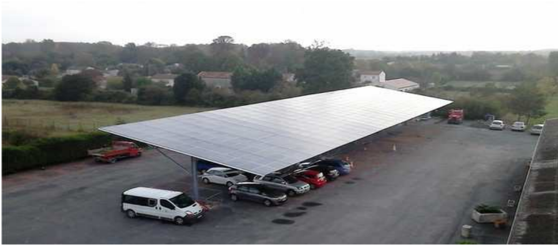
Ombrière photovoltaïque – P= 99,36 KWc - parking ateliers intercommunaux- Fossemagne
